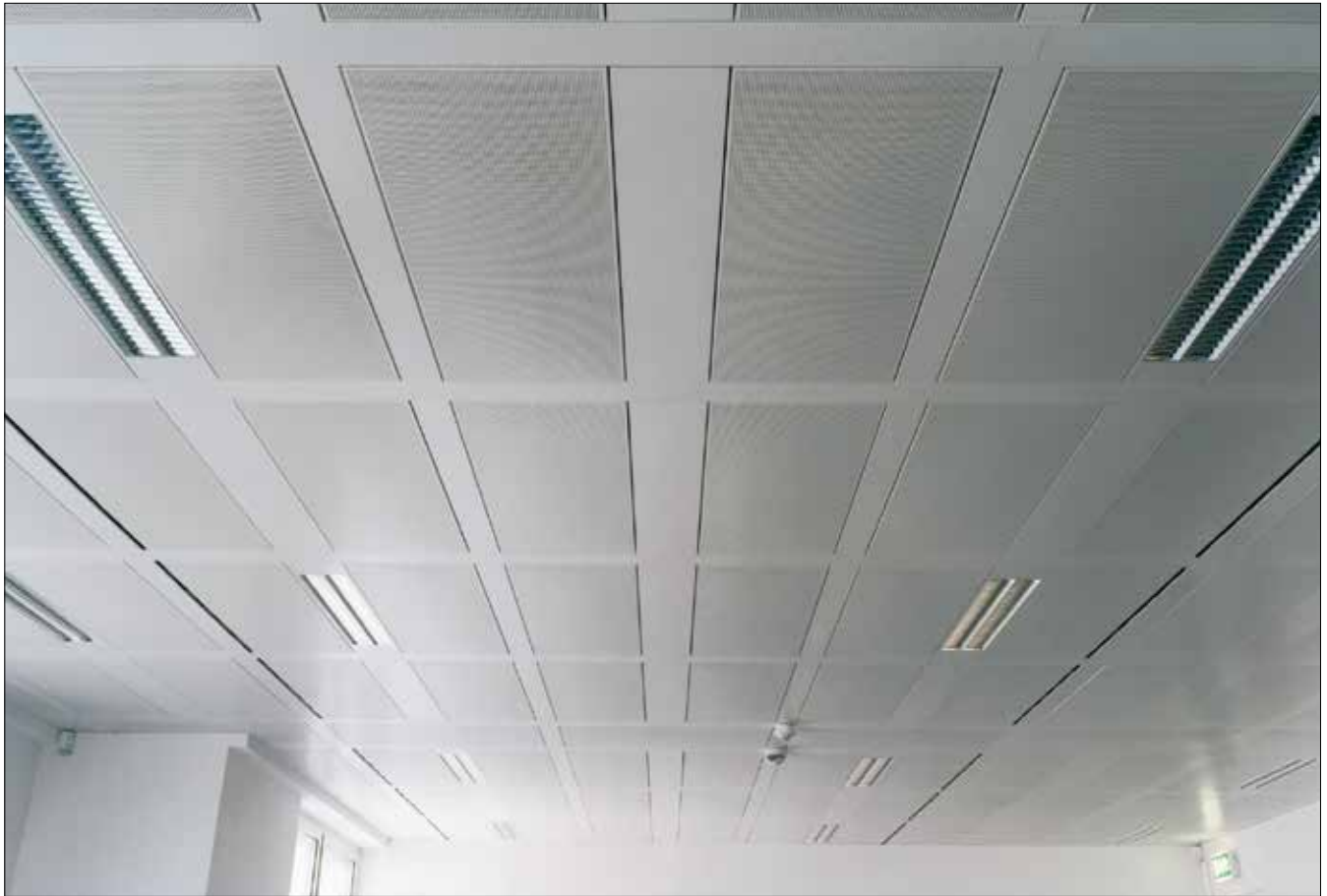
Cross bandraaster ceiling system, without junction boxes, using three panels per module.
