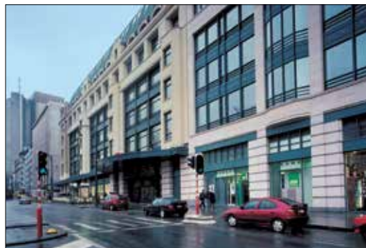
Fortis City Centre, 21.000 m 2 Brussels, Belgium
