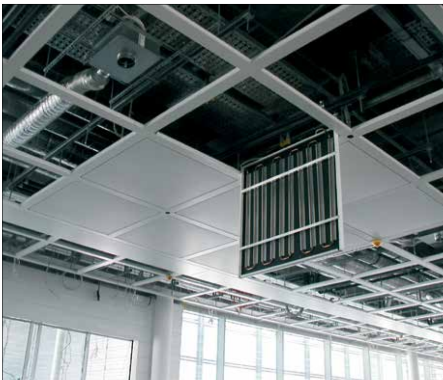
Chilled ceiling panel system containing copper cooling elements. Individually accessible without the use of tools, using a simple 'push & release' system.
