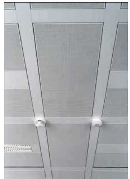
Intermediate cross bandraaster ceiling system; module 600 x 1200mm using one panel per module.
