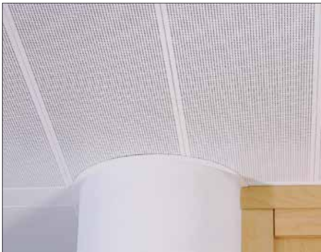
Detail showing column ring.
