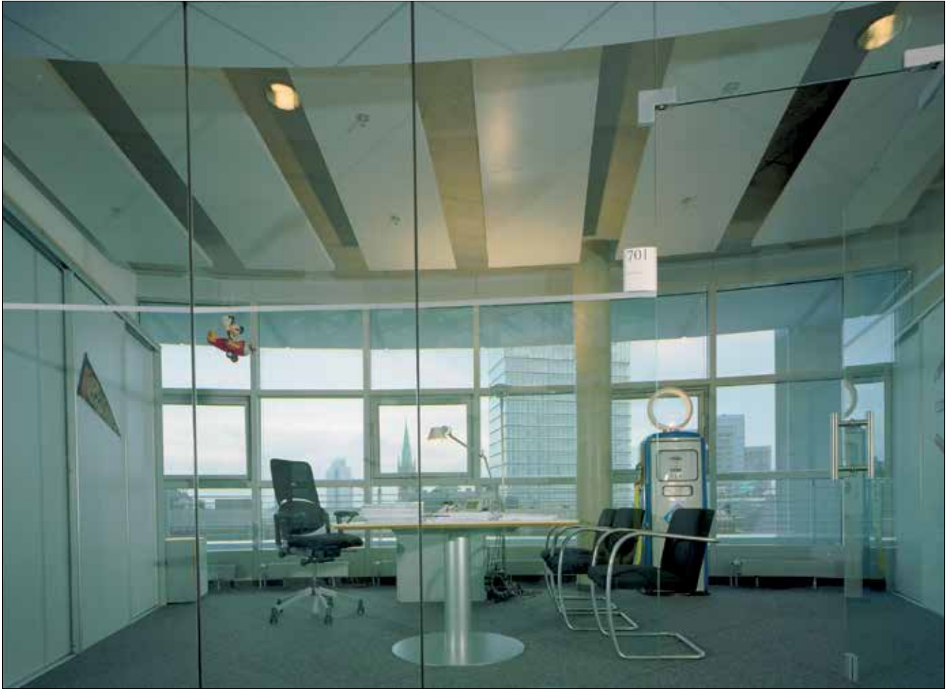
Trapezoidal ceiling islands in an elliptical shaped building.
