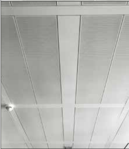
Cross bandraster ceiling system; module 1800 x 1800 mm.
