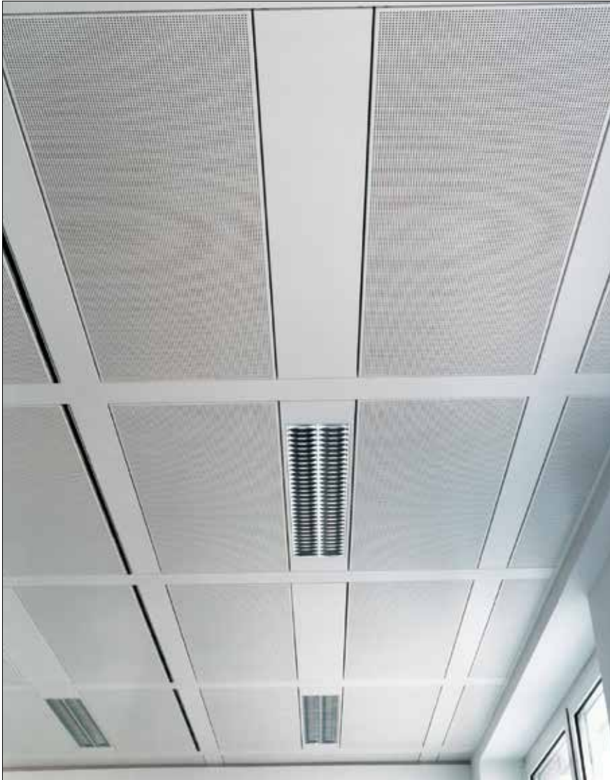
System QB with cross bandraster using connector bracket
