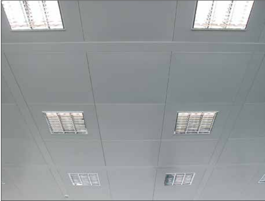
Cross bandraaster ceiling with 9 panels per module.
